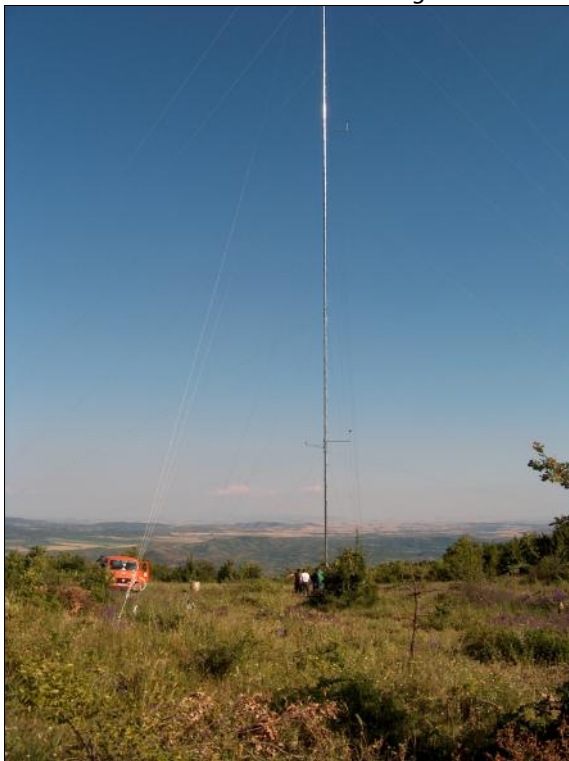
Picture 2 – Bogdanci Site – Measurement Mast
