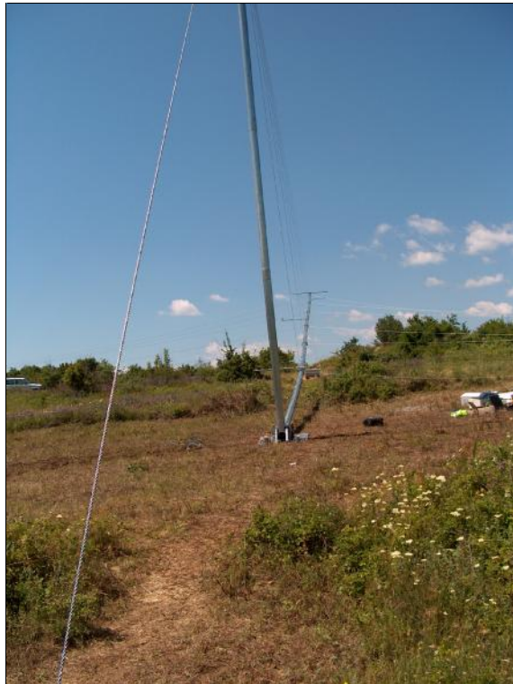
Picture 1 – Bogdanci Site – During erection of the mast
